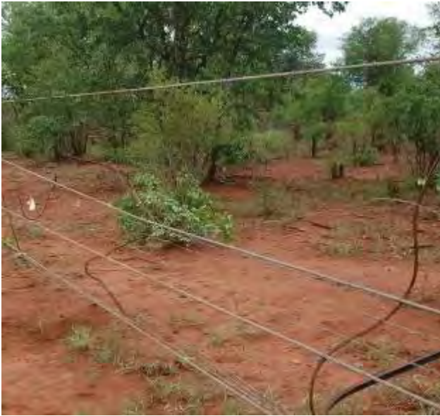
13mm cable fencing damaged by elephants at Kruger National Park © Ken Ferguson
